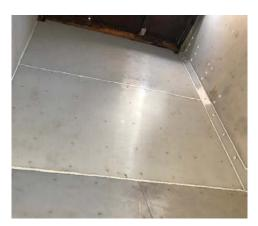
K-Slide UHMWPE Low Friction Liner features unique properties that deliver a low co-efficient of friction, superior abrasion and corrosion resistance. The UHMWPE low friction liner is light weight and easy to work with. However, they cannot be used in continuous service above 85 degrees C, or where they are subject to large or sharp feed with high energy.
